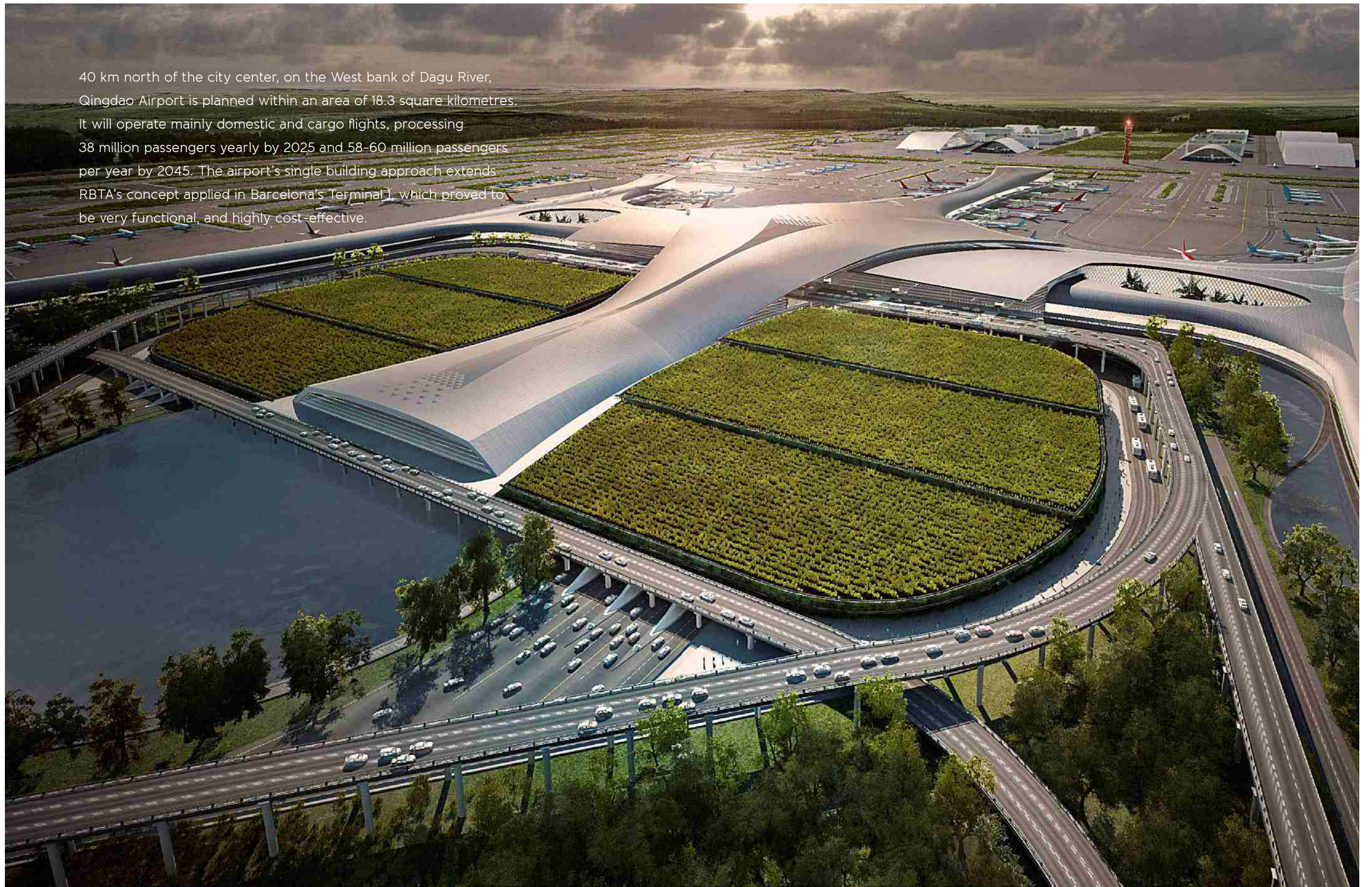
Qingdao New Airport, China
