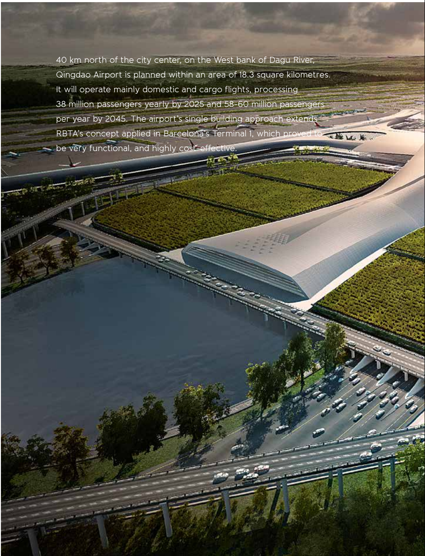
Qingdao New Airport, China
